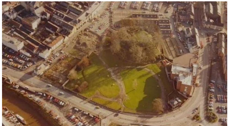
Library site under demolition/excavation. Top right: the cattle market buildings were still in use. (North Devon Local Studies P251885)
